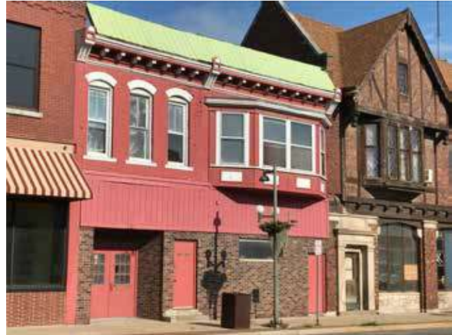
121 North Market Street, Oskaloosa, IA
